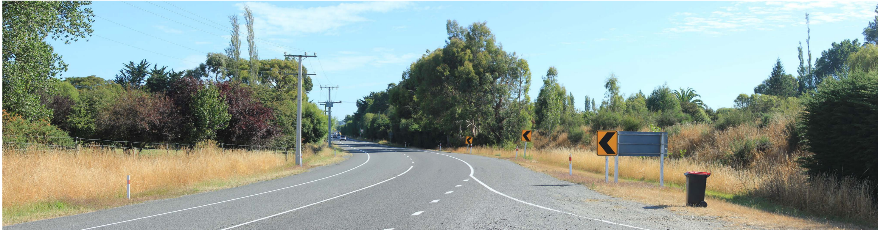
Site Photograph 7: Looking to the north along SH1 from Preece Road.
