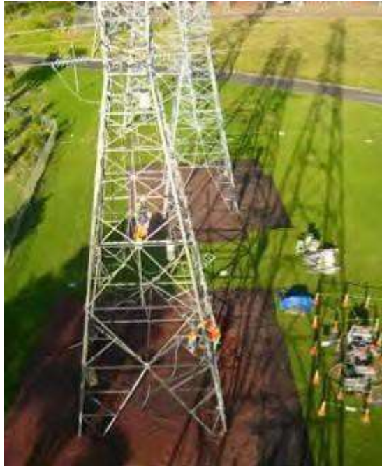
Figure 6: Abrasive blasting in area with no under-build
