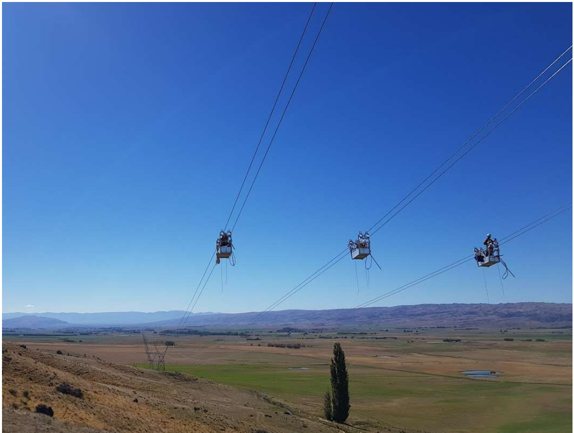
Figure 9: Depiction of conductor trolleys in use on a Duplex conductor
