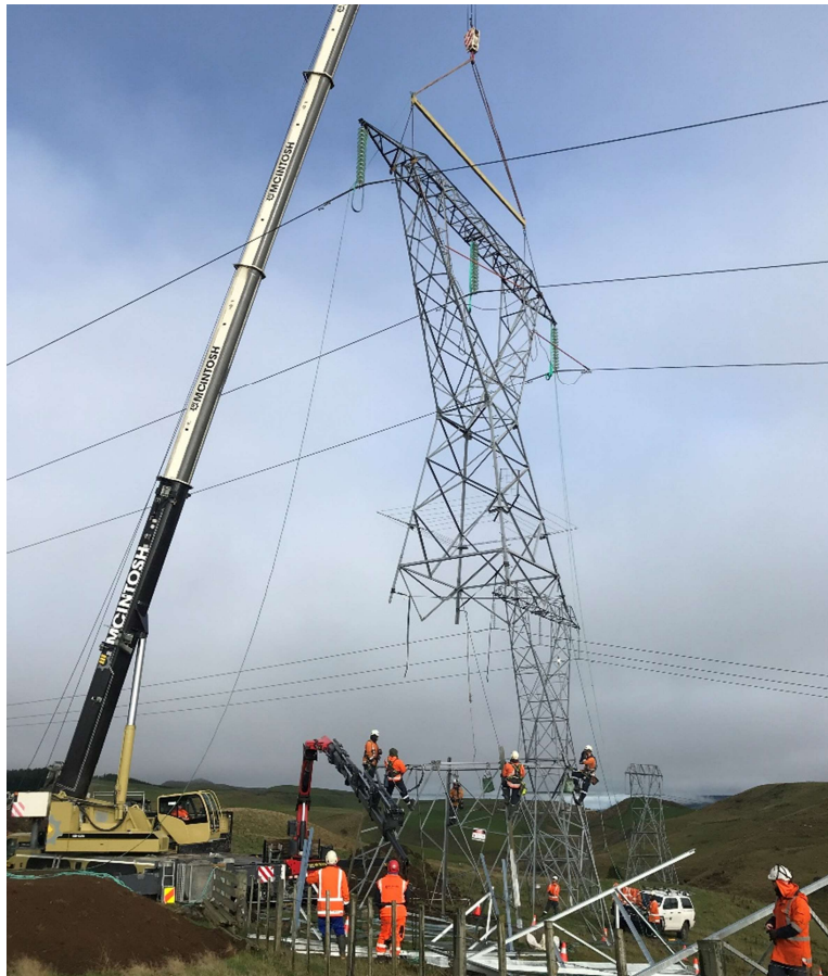
Figure 8: Parallel Body Extension being installed on the BPE-WRK-A line
