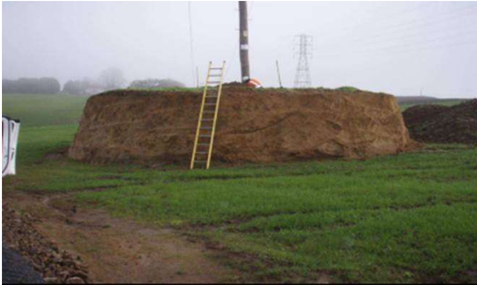
Figure 20: NZECP34 compliant earthworks around a pole on the ARI-HAM-A line
