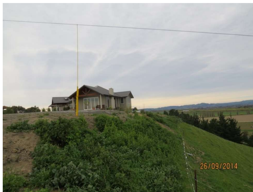
Figure 29. Hastings ground clearance violations
