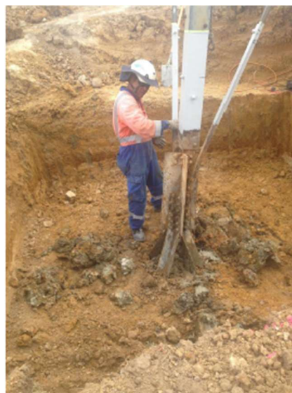
Figure 2: Land disturbance during foundation replacement
