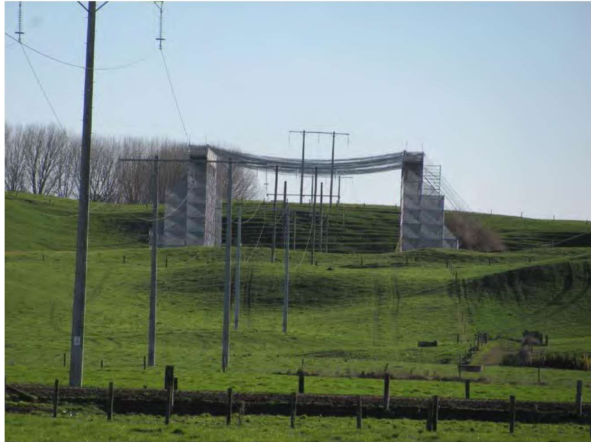
Figure 10: Scaffolding protection structure for stringing
