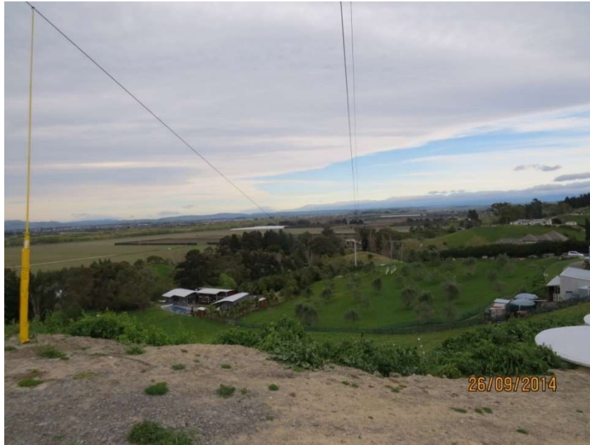
Figure 1. Hastings ground clearance violations
