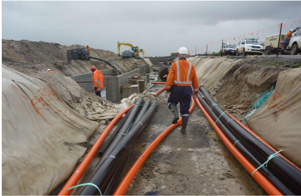
Figure 11: 110kV underground cable installation
