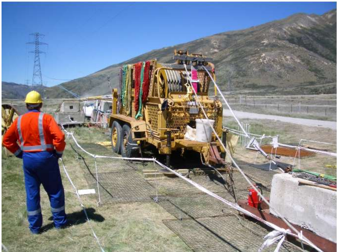
Figure 14: Reconductoring site from an ISL-KIK-B stringing project
