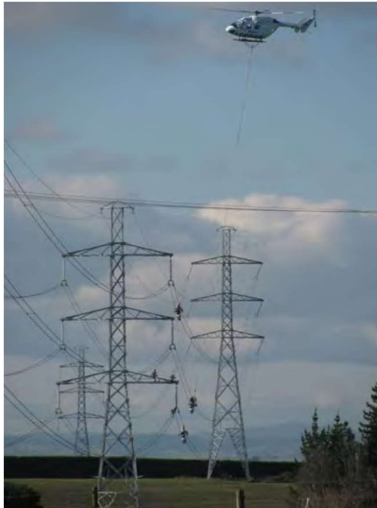
Figure 7: Maintenance work being carried out using helicopters
