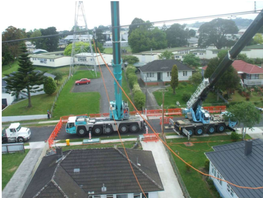
Figure 17: Reconductoring in an urban setting
