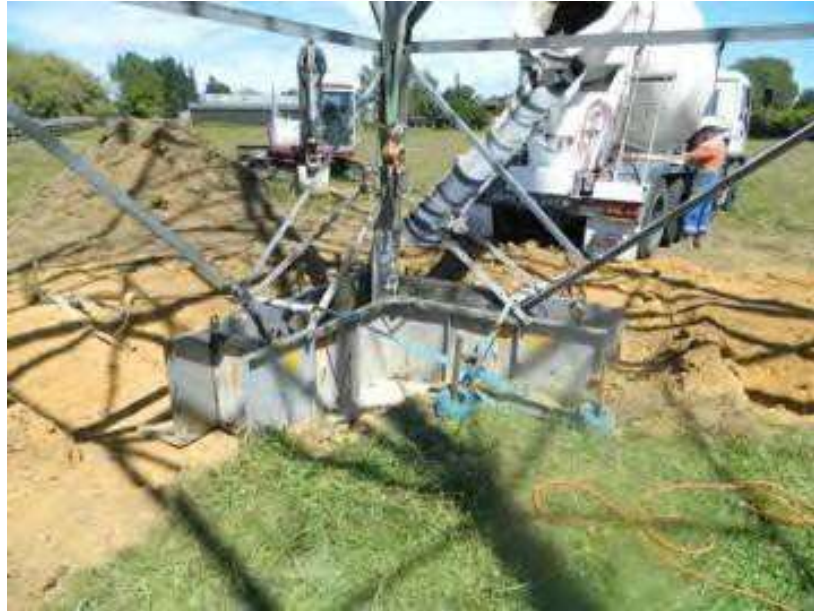
Figure 1: Grillage foundation replacement
