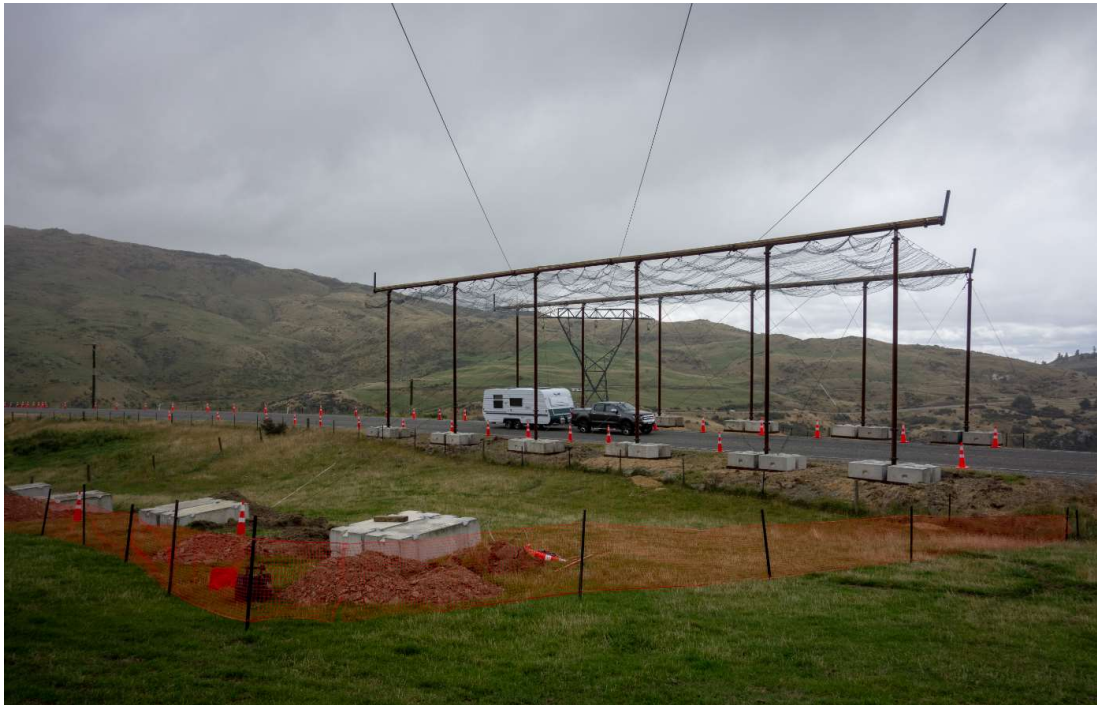
Figure 15: Hurdles installed to mitigate potential conductor drop during wiring
