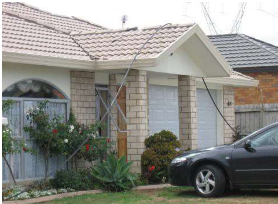
Figure 23: A conductor drop
