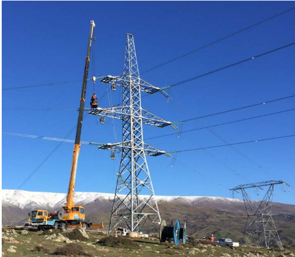
Figure 13: Crane being used for conductor stringing
