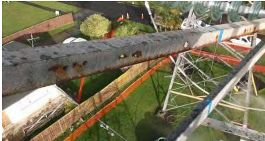
Figure 3: Tower Corrosion
