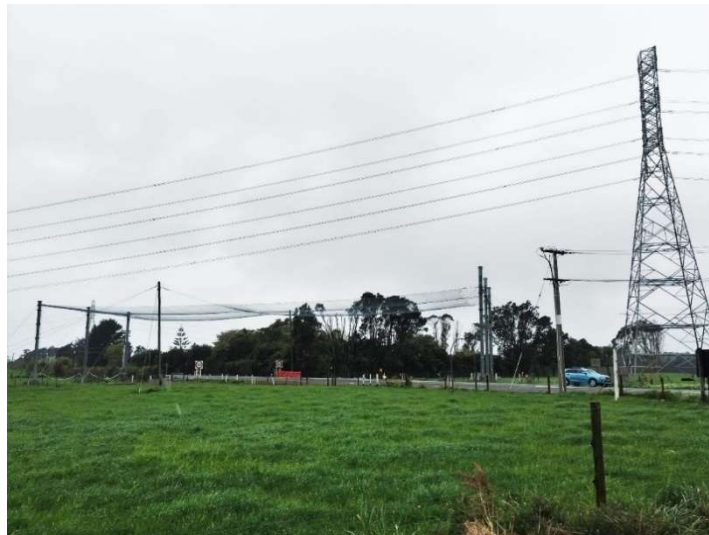
Figure 16: More substantial hurdles installed to mitigate potential conductor drop during wiring
