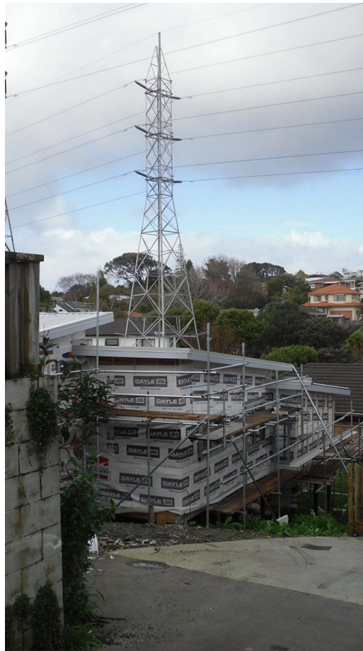
Figure 30. Dwelling blocking access to tower
