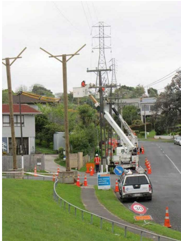
Figure 12: Removal of copper conductor on Pakuranga- Penrose A line
