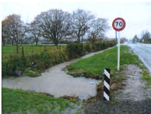
Figure 1 Water race along the eastern side of Lehmans Rd
