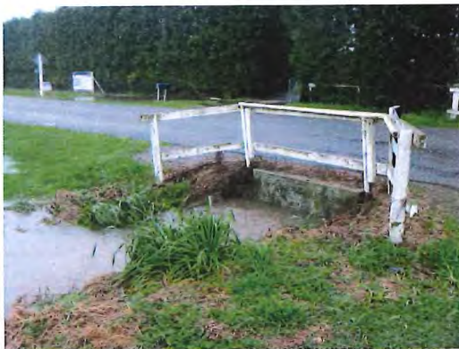
Figure 3 Culvert beneath Lehmans Road
