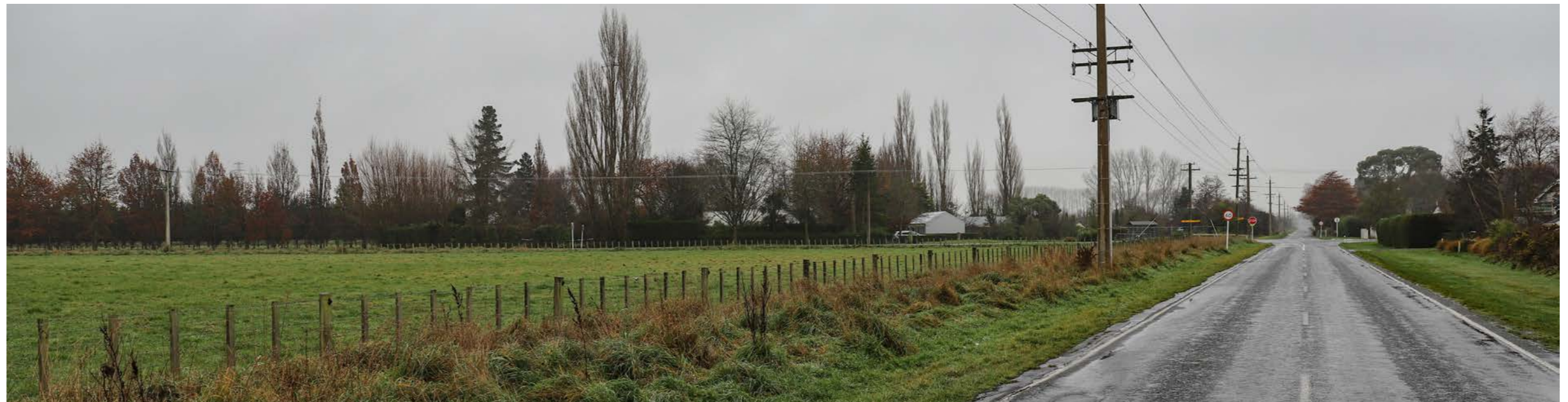
Viewpoint I2 - NE Bradleys Road Water Pumping Station
