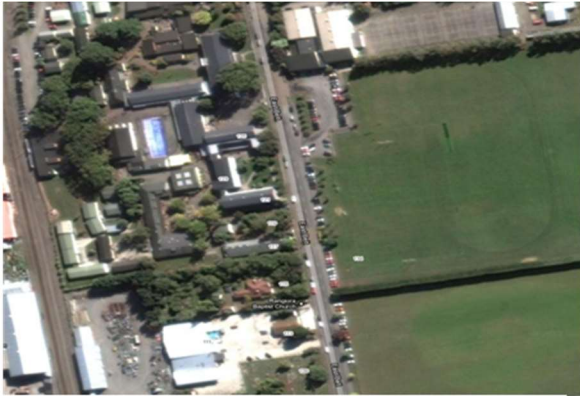
Rangiora Baptist Church, 111 East Belt Rd
