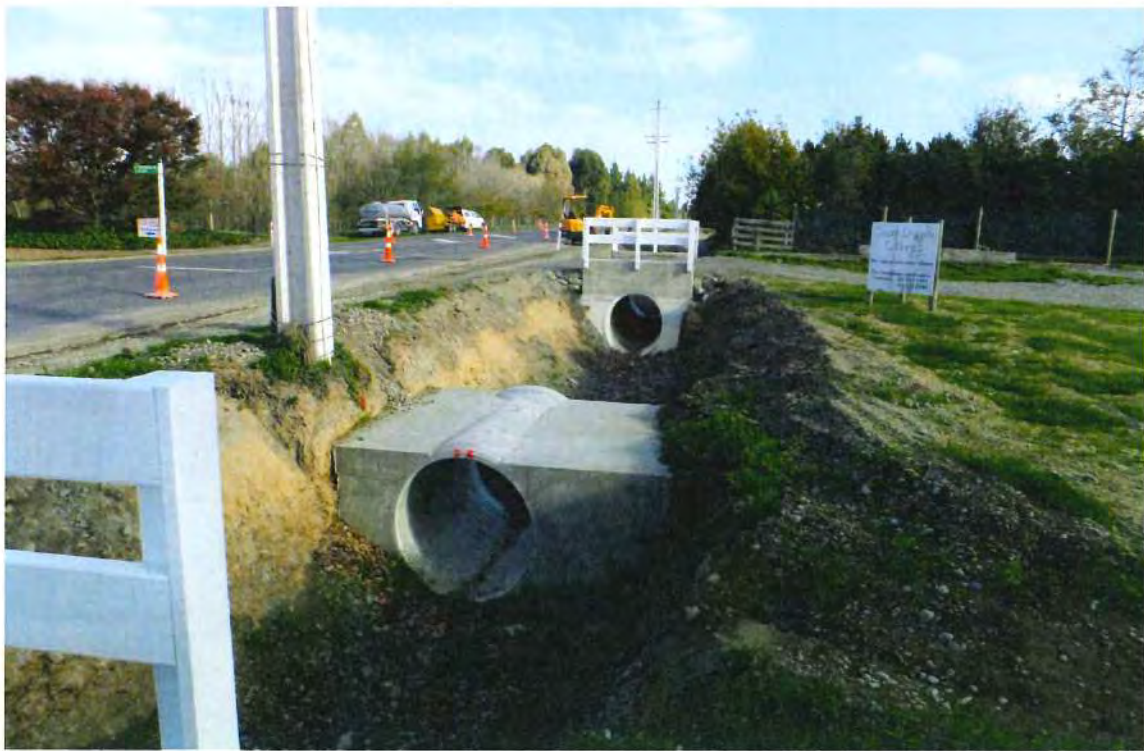
New flood mitigation works in the enlarged drain culverts along Bradley's Road.
