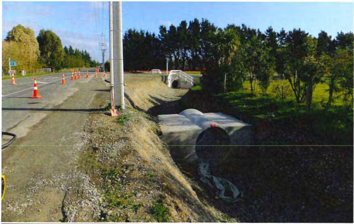
New flood mitigation works in the enlarged drain culverts along Bradley's Road.
