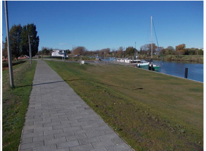
Figure 3: Stop bank, Kaiapoi River left bank (Kaiapoi)
