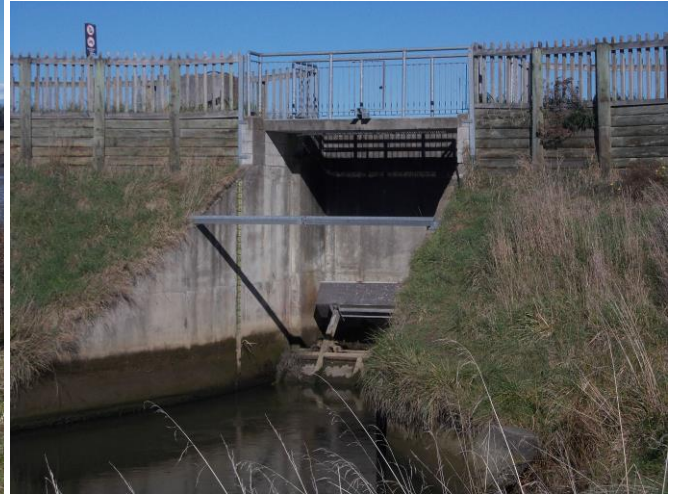
Figure 4: Stop bank, Ashley River right bank (Waikuku Beach) Figure 5: Gated outfall to Ashley River (Taranaki Stream)
