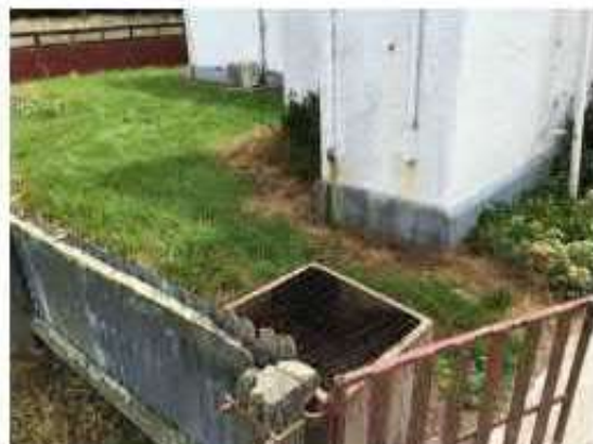
Figure 4: Concrete bin that appears to have been used to incinerate domestic rubbish. It is not known where potentially contaminated ash has been deposited.
