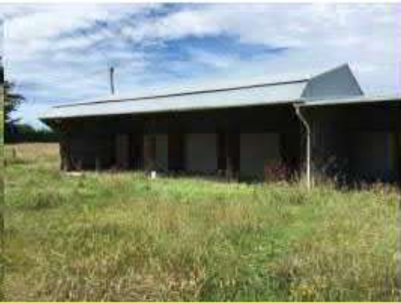
Figure 6: Horse stables, originally constructed pre-1940s, presumably as shearing shed.
