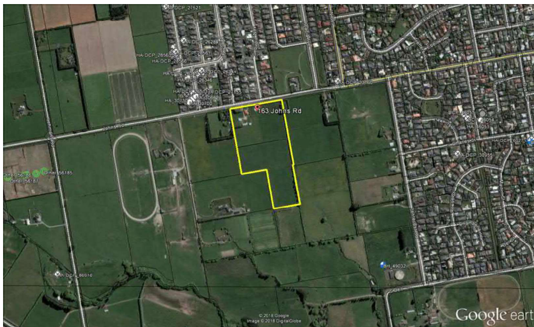
Figure 5: Plan of existing geotechnical deep investigation. Note the recent deep test is located around 400m southeast of the site.
