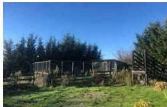
Photo 4. Cattle yards and garden shed
