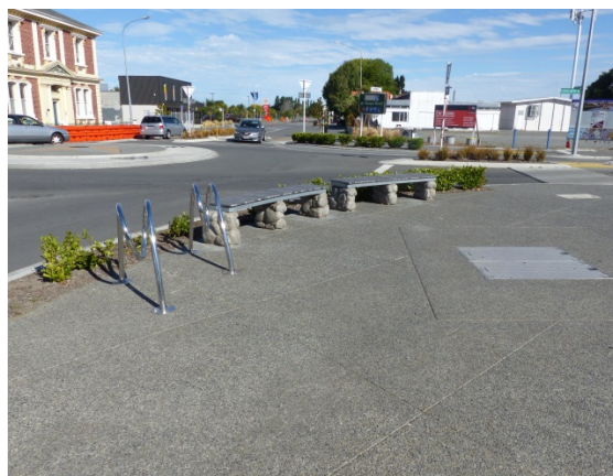
Photo 3: Street works at Intersection of Williams / Charles Streets
