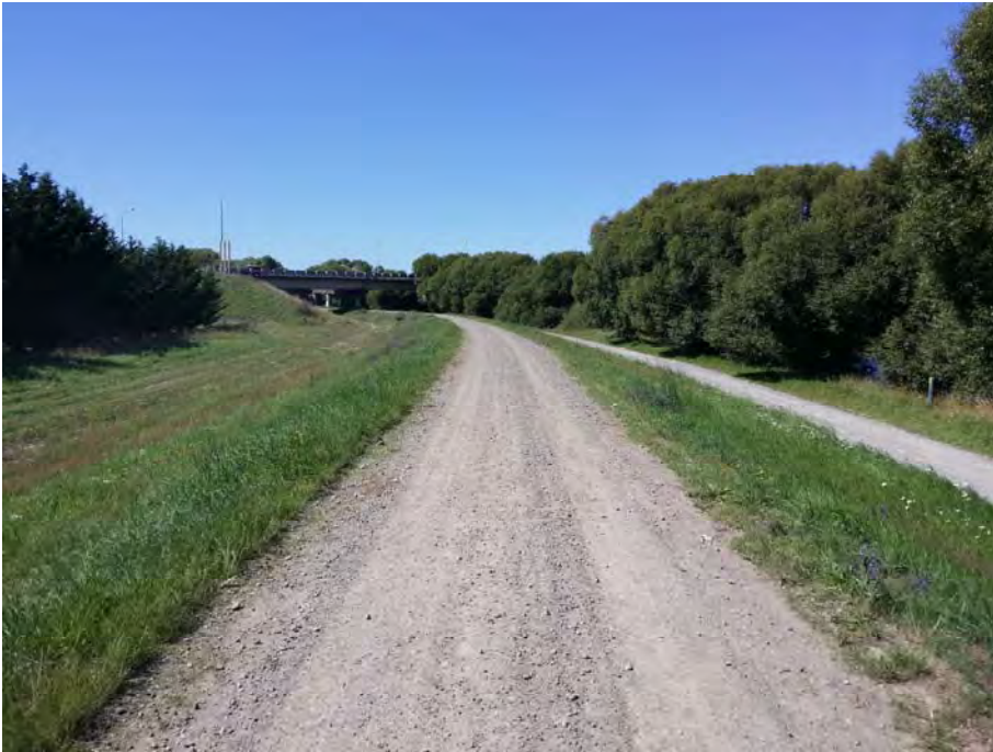
Kaiapoi River stopbank
