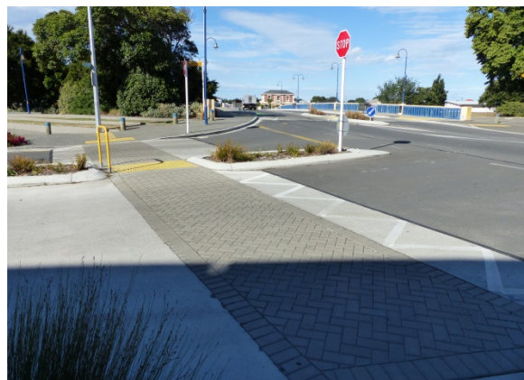
Photo 9: Street works at Intersection of Williams Street and Raven Quay
