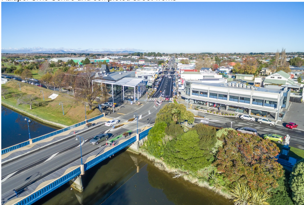
Photo 1: Aerial looking south down Williams Street showing the new Ruataniwha Kaiapoi Civic Centre and completed street works
