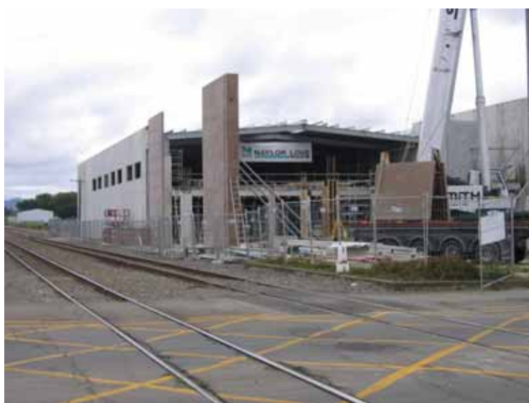
Rangiora Bakery building under construction
